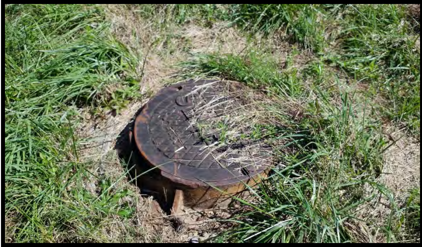
View of sewer cover on PA-2.
