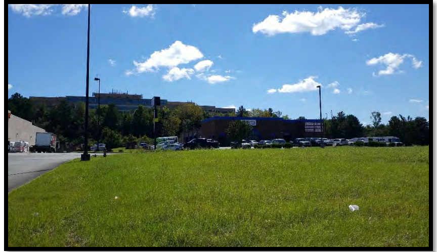
View of PA-3 and adjoining property to the east.
