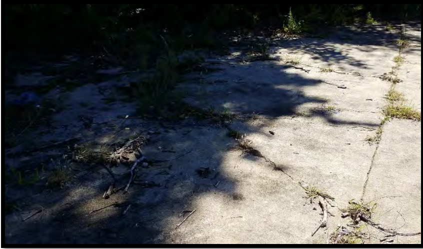
View of PA-6 concrete slab.
