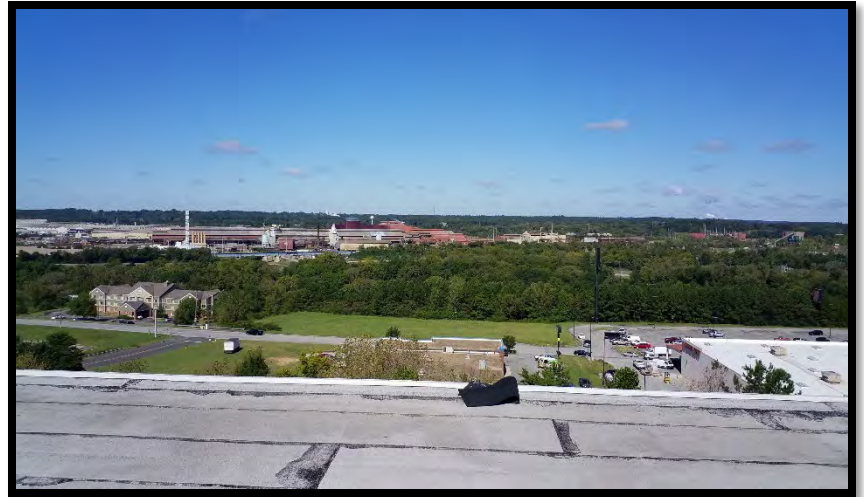
View on roof facing PA-3.
