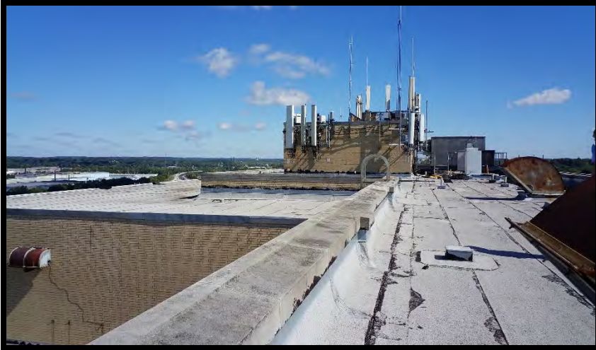
View on roof.
