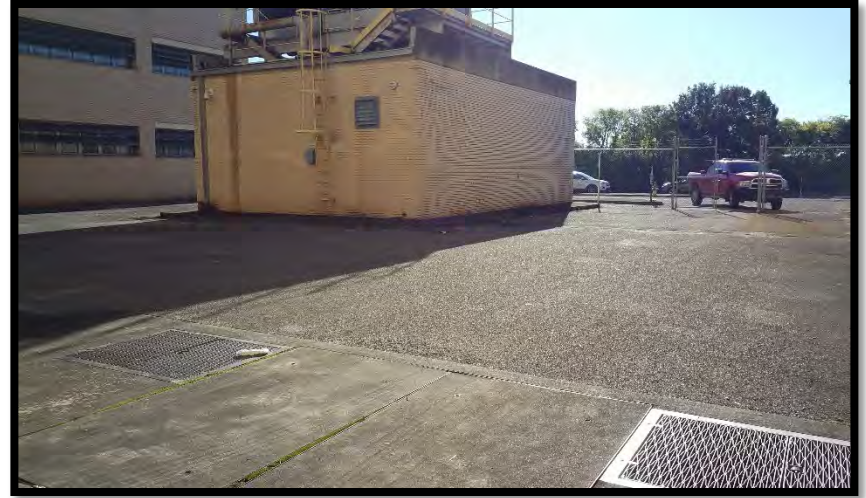
View at the east side of the building.
