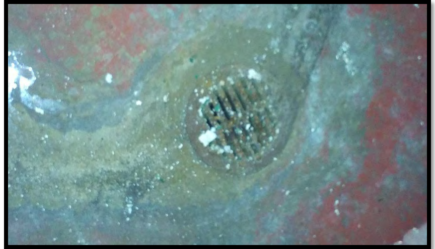
View of floor drain in basement.
