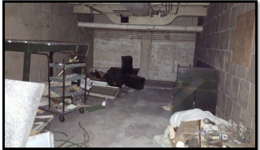
View of vault interior.
