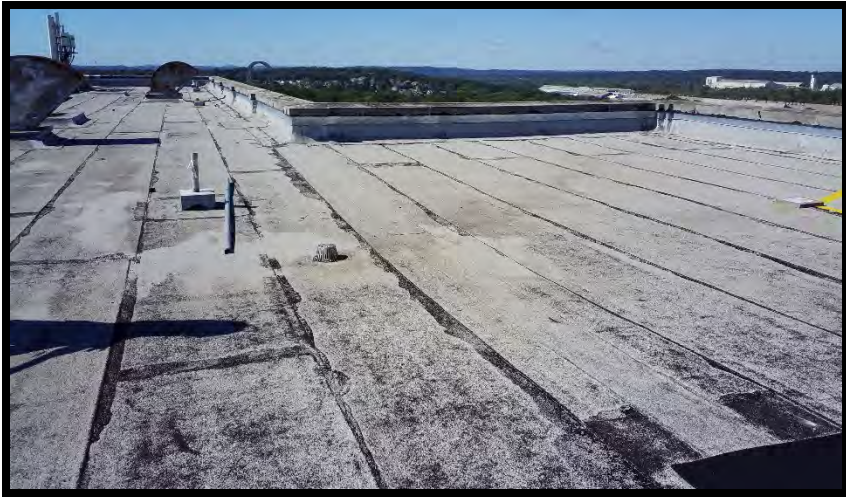
View on roof.
