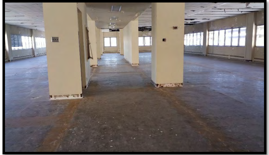
View of 2nd floor room.
