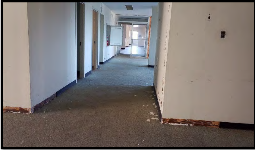
View of 2nd floor offices.
