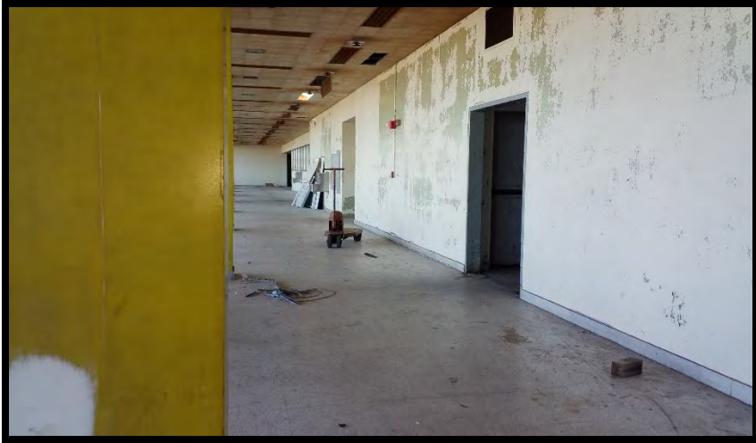
View of cafeteria.
