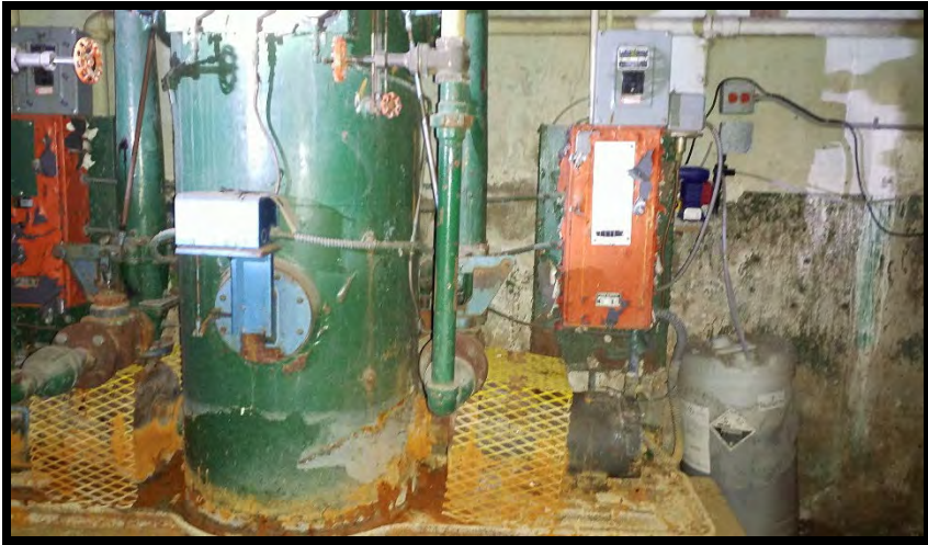
View of differential pump.
