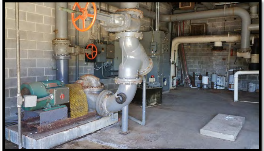
View inside small building to the east of the main building.
