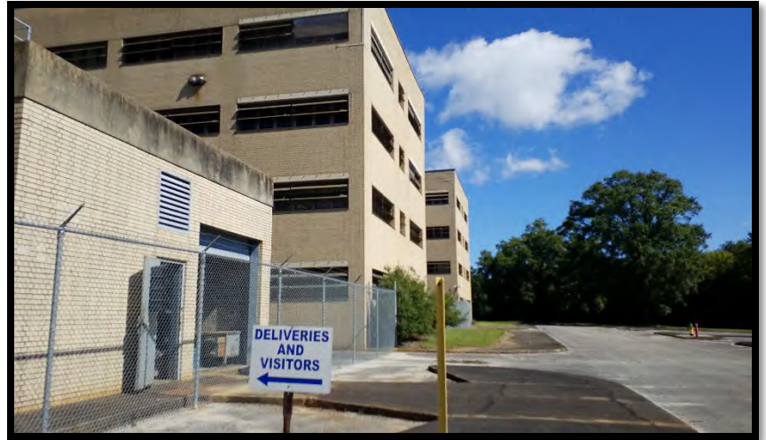
View along the east side of the building, facing north.
