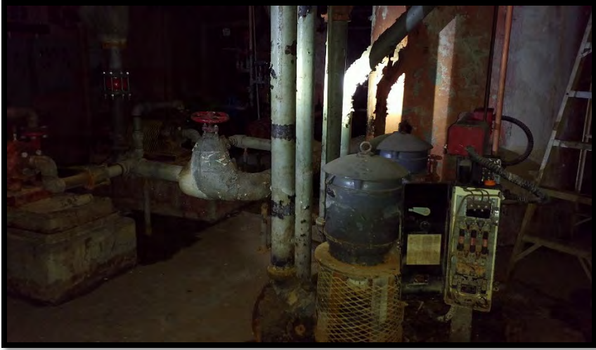
View of basement.
