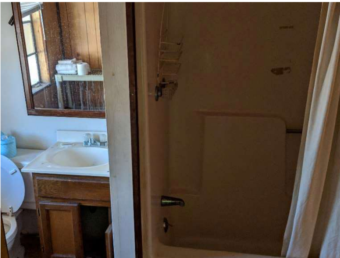
Photo #5 View of typical bathroom in rooms 121-140
