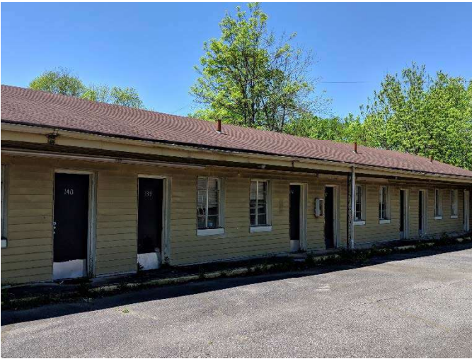
Photo #3 View of 133-140 building
