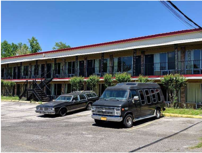
Photo #1 View of front of 2535 House
