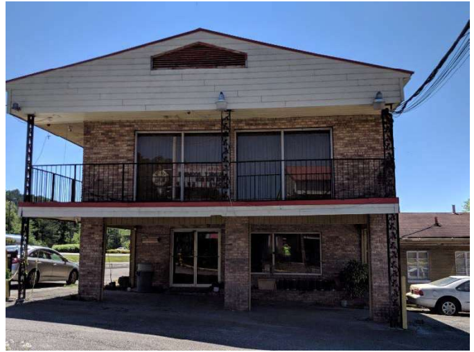
Photo #2 View of side of Office Building
