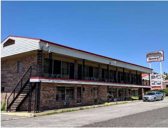
Photo #1 View of front of Office Building
