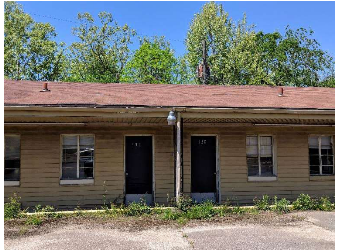
Photo #2 View of 129-132 building
