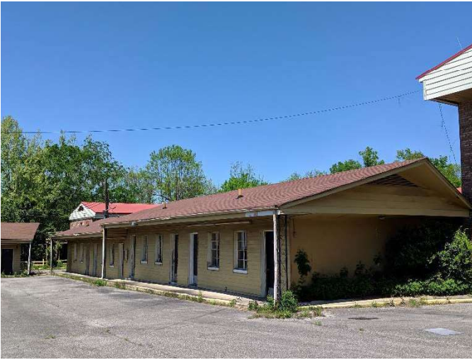
Photo #1 View of 121-128 building
