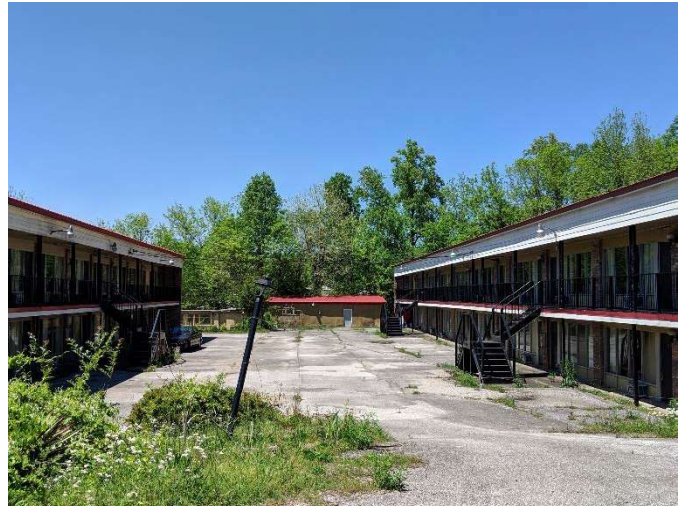
Photo 2 View of Storage Building at the north end of rooms 151-160 & 251-260
