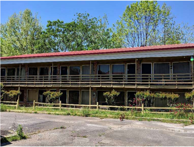
Photo #1 View of front of 2505 House
